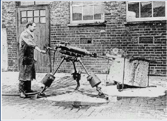
Silent sonic gun using compressed liquid and an explosive charge.
